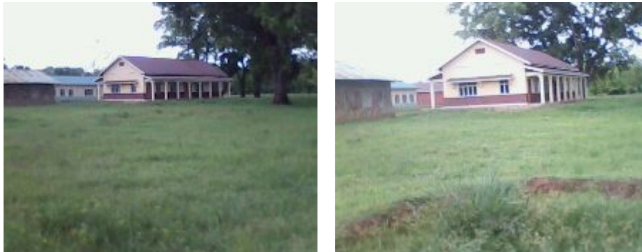
Amadi Rural Development Institute (ARDI) undergoing rehabilitation
