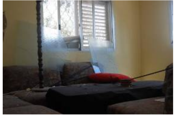
Home in Sderot damaged by rocket fire (Hamutal Ben-Shitrit for www.sderotmedia.co.il , June 24).
