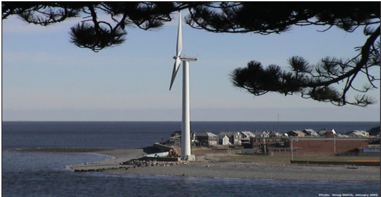
Figure N: 600 KW Turbine Developed, Financed, and Installed by the Hull Municipal Light Plant in 2001 on the Coastline beside its Elementary School.
