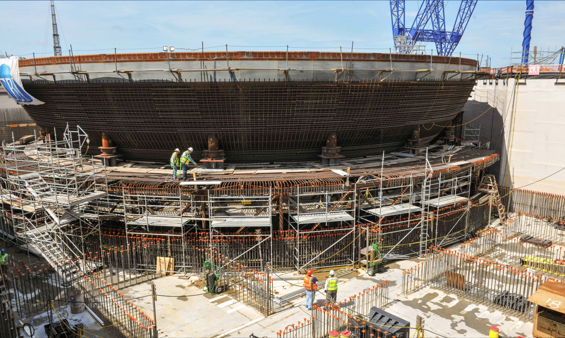
Plant Vogtle Unit 3 containment vessel bottom head inside nuclear island
