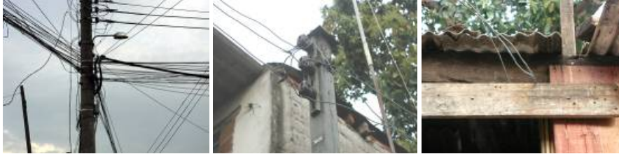
Figure 2 – Students’ documentation of the dangerous illegal energy connections, which they hoped to transform through an educational pamphlet to teach the population to make safe illegal connections.
