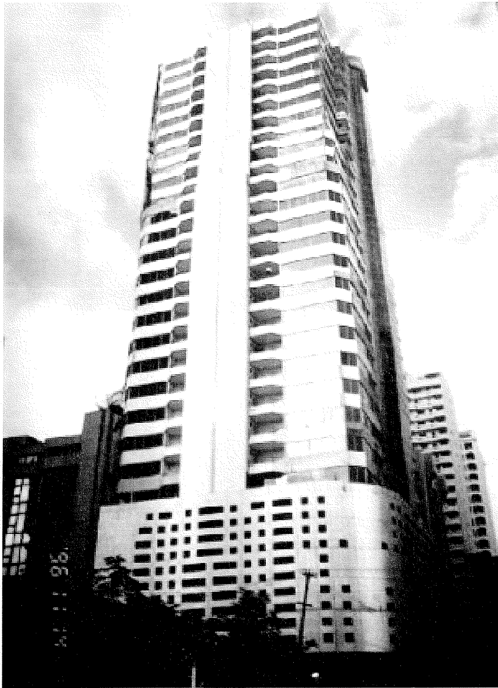
Figure 4. 30-story “Chatham Building”
