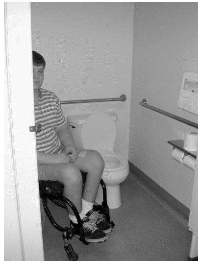
Figure 6.12: Wheelchair user access to the women's toilet.
