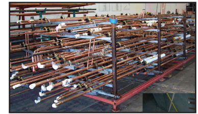
Shop Pipe Assembly - T&S
