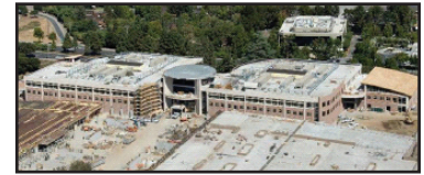
Project under construction
