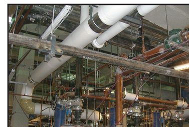
Piping installed per detailed 3D coordination model
