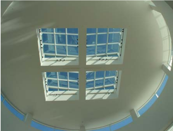
Fig. 14 – Getty Museum’s Computer-controlled Skylight is similar to those in the Montage Laguna Beach Hotel. They are installed in various galleries that change their angles to let a different amount of light in as the outside conditions vary, saving money and increasing the amount of natural sunlight in the room.
