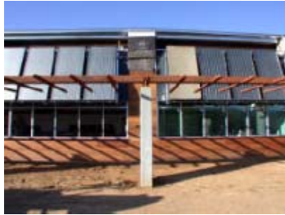
Figure 6: The photovoltaic panels not only generate solar heat, but also provide shading for the north side of the building during the summer months, reducing the internal temperature of the building.
