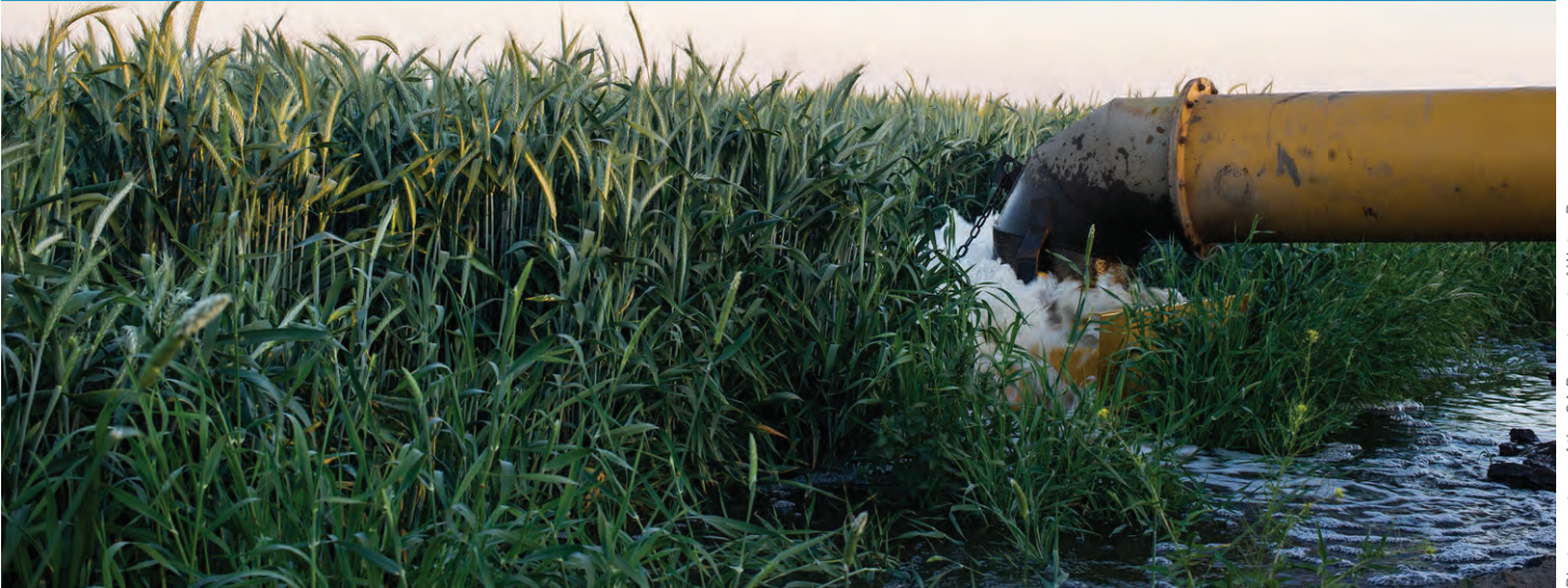
Photo courtesy of the CA Department of Water Resources
