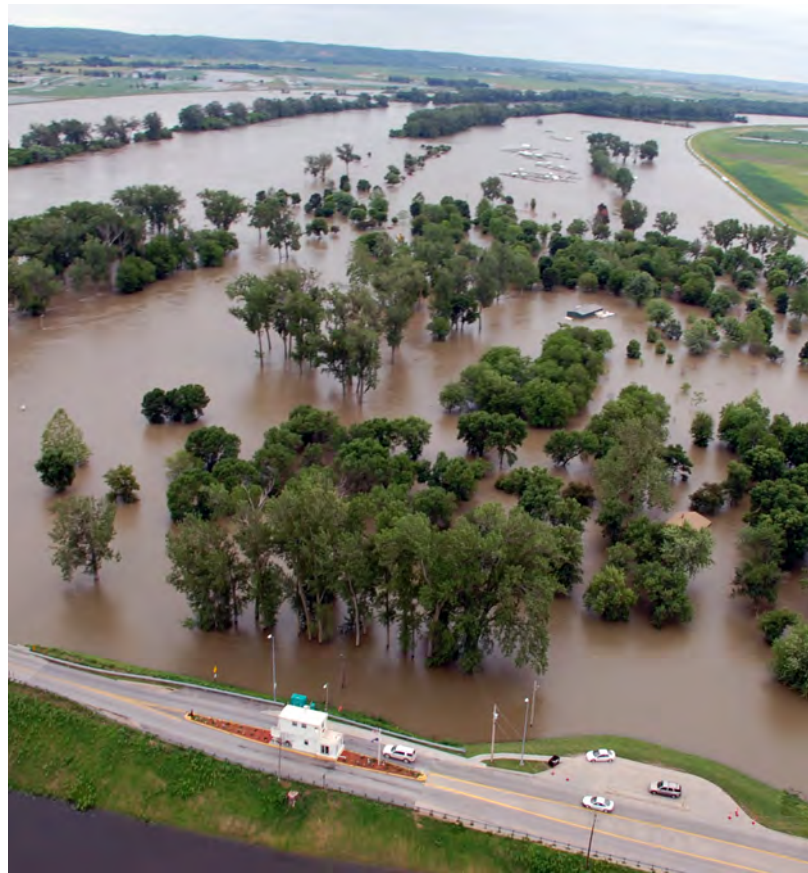
Bellevue, NE—The flooding Missouri river captures more land around the Bellevue Bridge. Access roads to the Marina are impassable. Courtesy of FEMA
