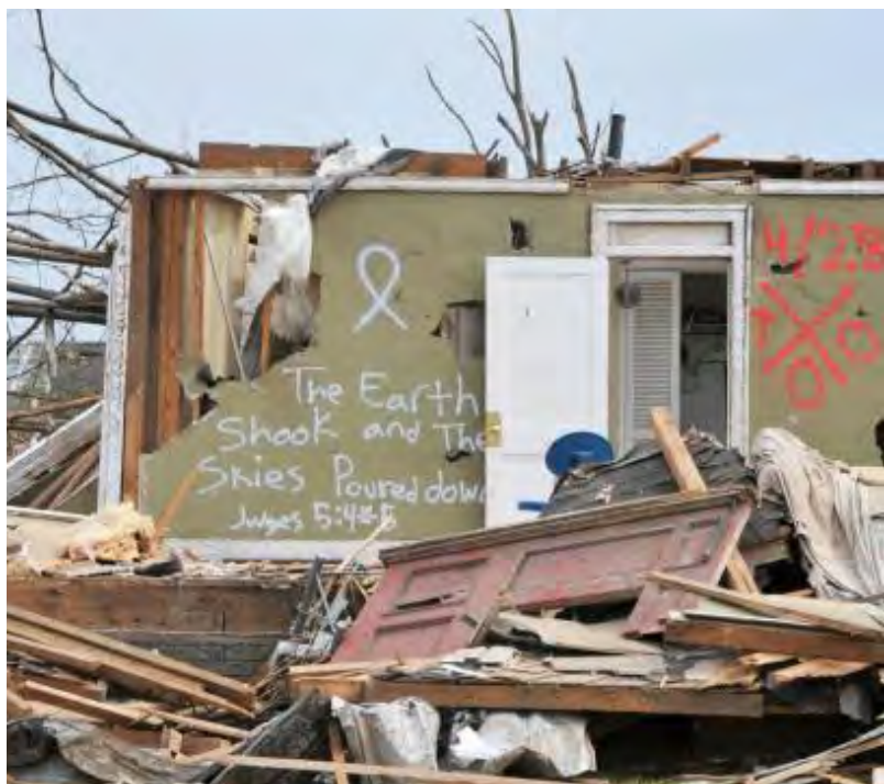
Tuscaloosa, AL tornado aftermath in 2011. Courtesy of FEMA
