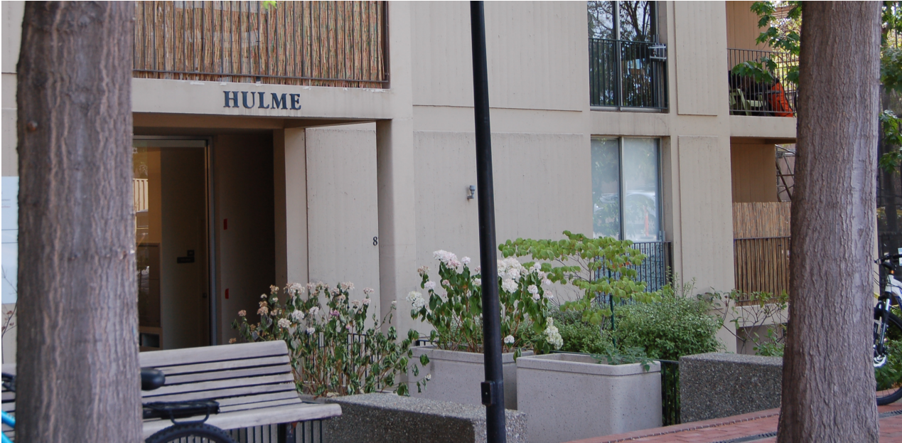
A fire sprinkler system retrofit in the Hulme Midrise will be fully installed by the end of the summer, 2014.
