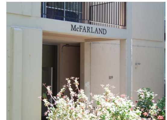
McFarland midrise will be fully sprinklered by the end of summer 2013
