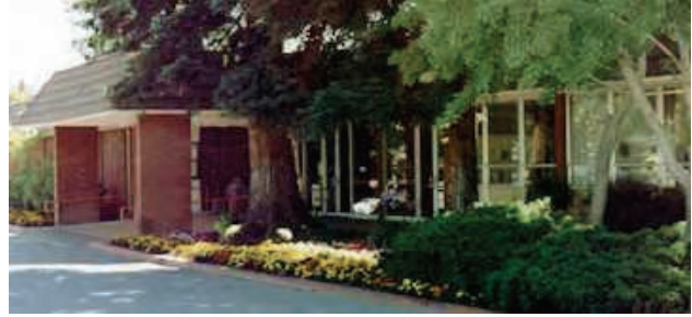
Community Activities Building 1400 Roosevelt Avenue Redwood City, CA 94061
