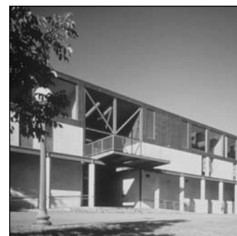
CHARLES B. THORNTON CENTER FOR ENGINEERING MANAGE- MENT 379 Santa Teresa Street Architect: Tanner Leddy Maytum Stacy Landscape Architects: Walker/Johnson and Partners Completed: 1994
