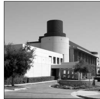
MEDICAL SCHOOL LAB SURGE/ LUCAS MAGNETIC SPECTROSCOPY CENTER 1201 Welch Road Architect: Stone, Marriaccini, Patterson Landscape Architect: David Gates and Associates Completed: 1992
