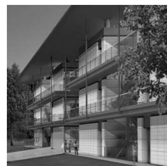
15 CLARK CENTER FOR BIOENGINEERING AND BIOSCIENCES
