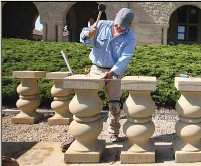
4. New, pre-cast balusters were installed in the original positions.
