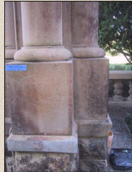
Redish brown stains on light posts were removed with Ferrous Stain Remover by Prosoco (above). Tests were first preformed to determine the workability of the product (right).
