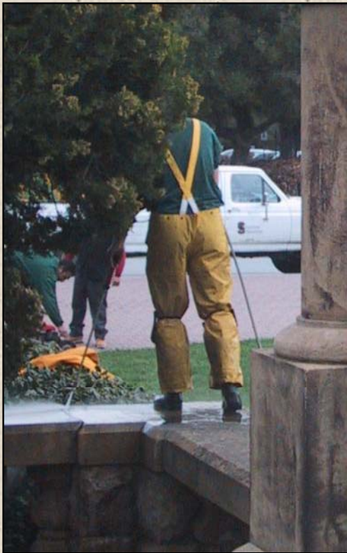
Power washing removed layers of dirt and biological growth.
