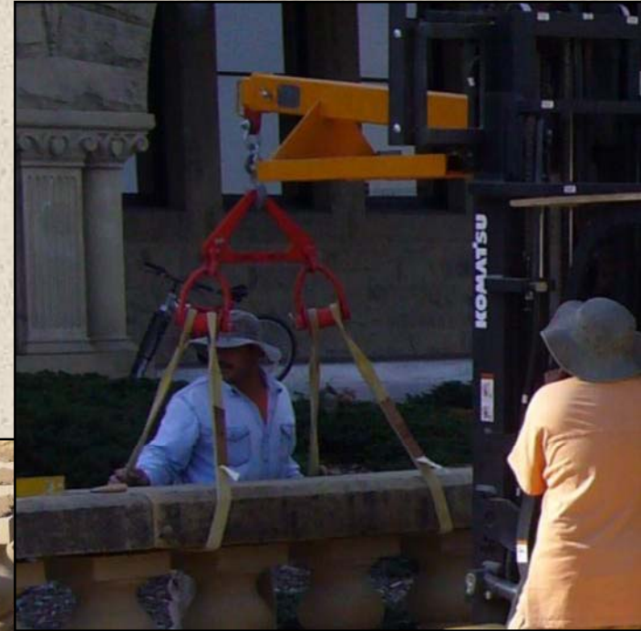
5. Top stones were replaced (above). Many top stones were curved slightly upwards on either end. Mortar thickness on top of the balusters (left) had to be adjusted to take this into account.
