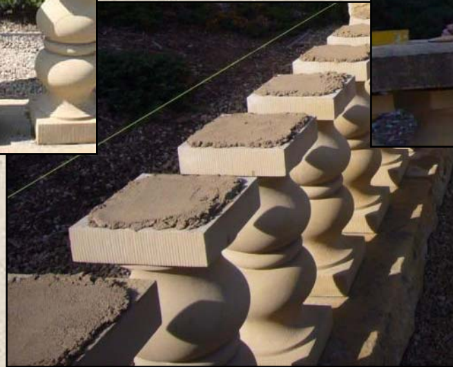
5. Top stones were replaced (above). Many top stones were curved slightly upwards on either end. Mortar thickness on top of the balusters (left) had to be adjusted to take this into account.
