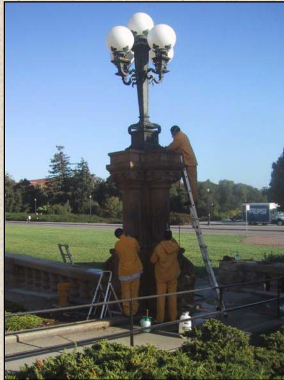
Redish brown stains on light posts were removed with Ferrous Stain Remover by Prosoco (above). Tests were first preformed to determine the workability of the product (right).
