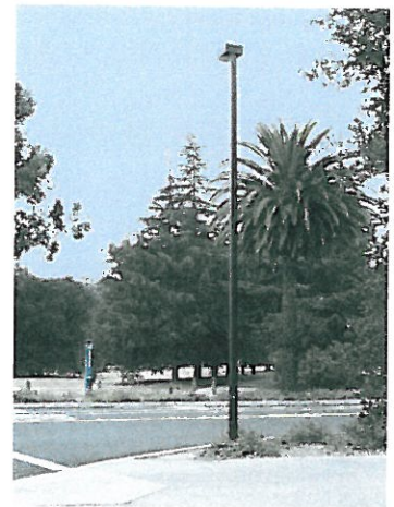
Intersection Light Fixture
