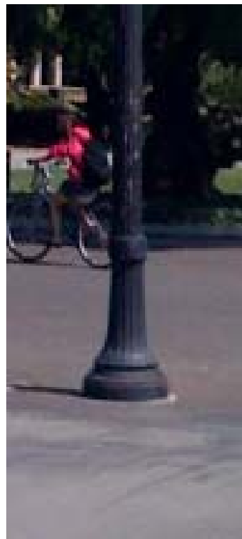
Detail of pole / base
