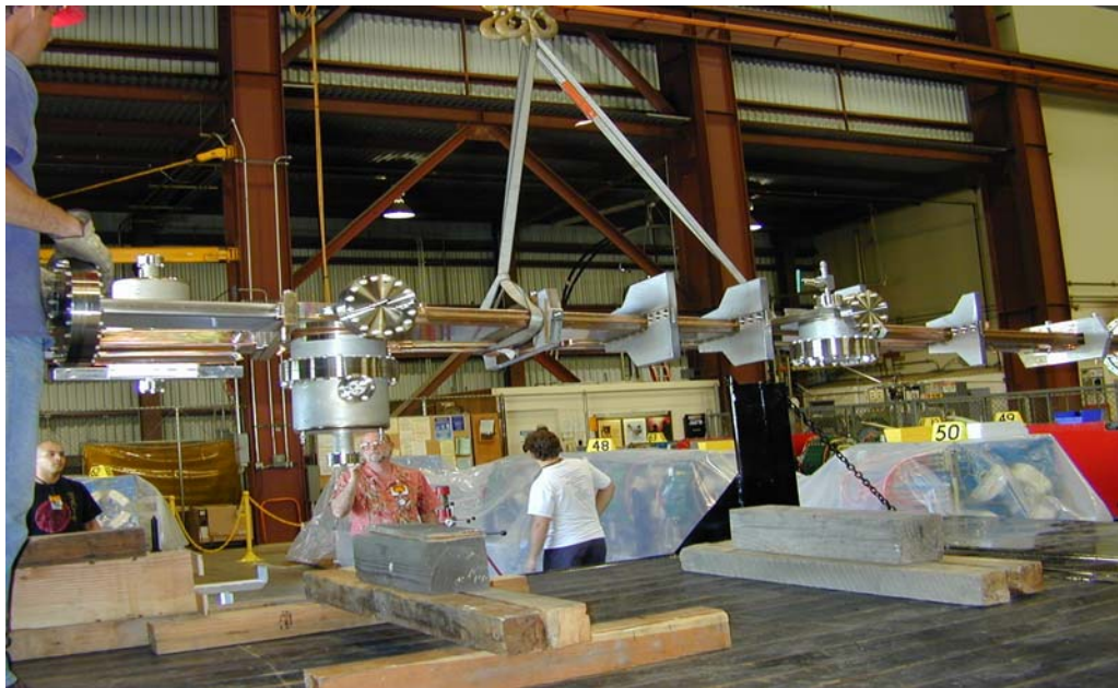
BM-1 Chamber Installation
