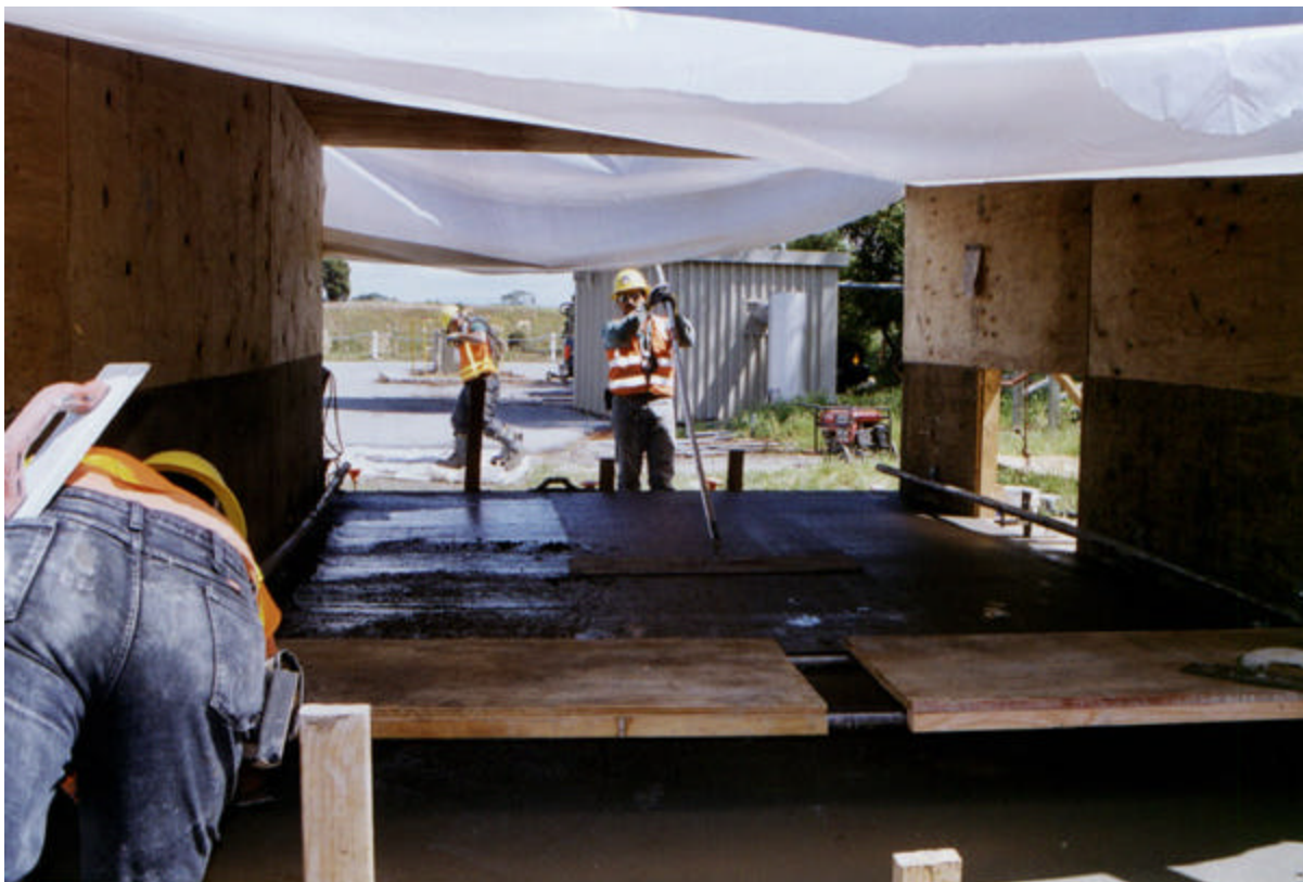
Construction of sample tunnel floor section in progress.
