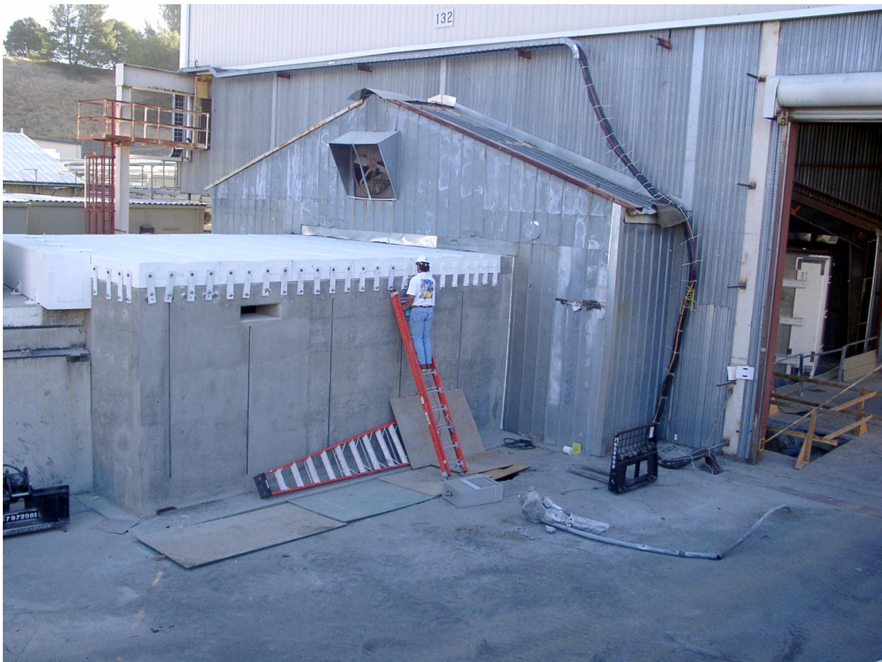
New Roof and Shielding for West Area
