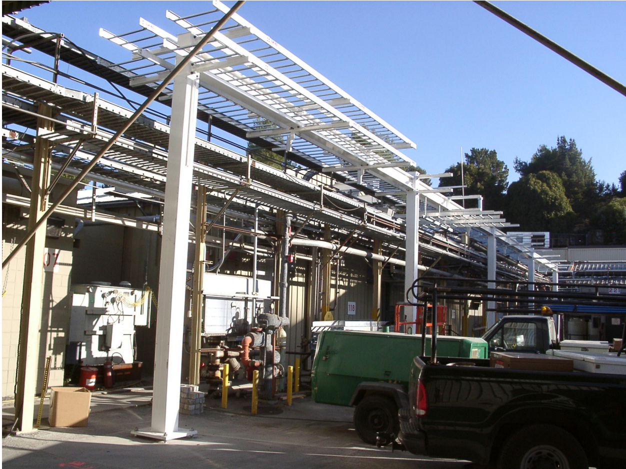
Installation of New Cable Tray System
