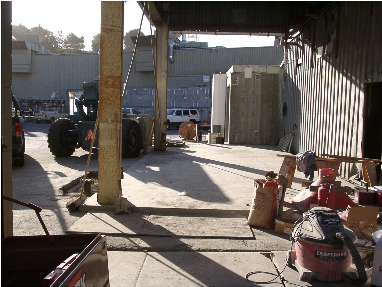
New Foundation for Klystron Enclosure
