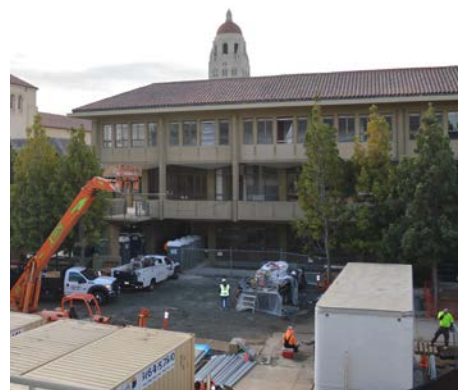
Construction at the new East Asia Library.
