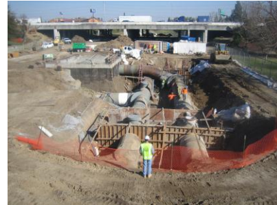
Mokelumne Aqueduct Interconnection Pipeline Project
