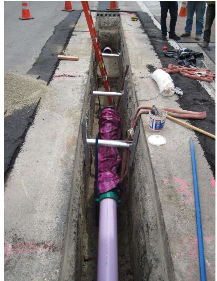
Alcosta Pipeline Installation, San Ramon
