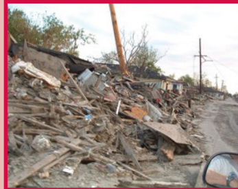
Massive Debris Pile for Grinding and Incinerations
