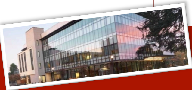
Photo: the new Stanford Neuroscience Health Center, opened in January 2016. Read more about it here .
