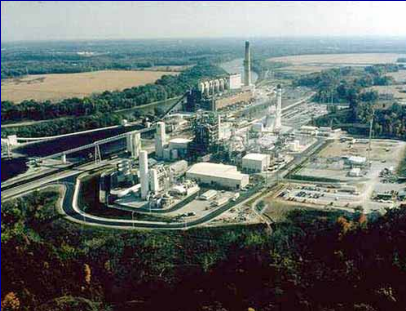
Wabash River Integrated Gasification Combined-Cycle Plant
