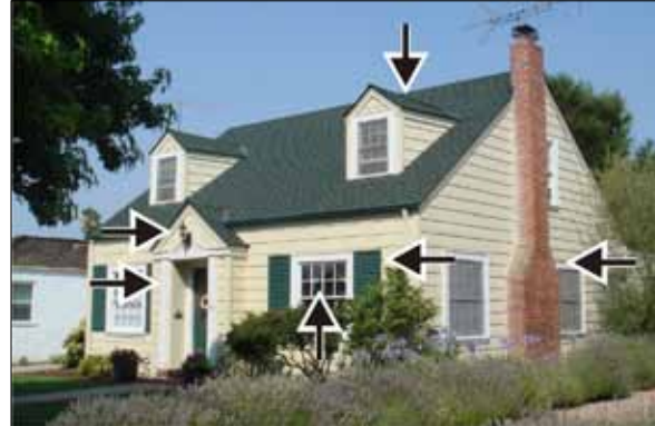
Dormers, wood shutters, divided light windows, carriage lights, and decorative door trim
