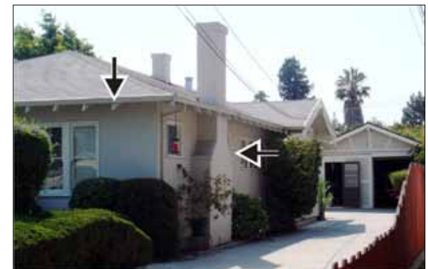
Exposed rafter tails and shaped chimney
