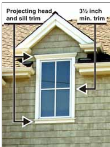
Wood trim with projecting heads and sills are common in traditional architectural styles
