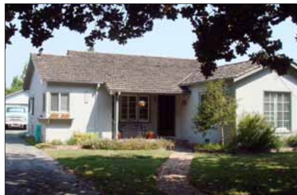
Entry under Roof
