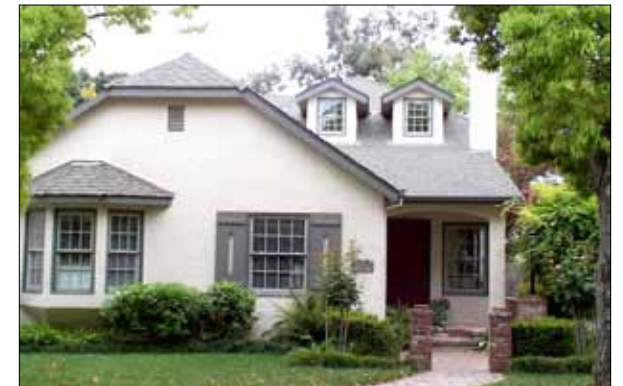
Good example of a bay window, shutters and matching windows adding rich detail to a home's street facade
