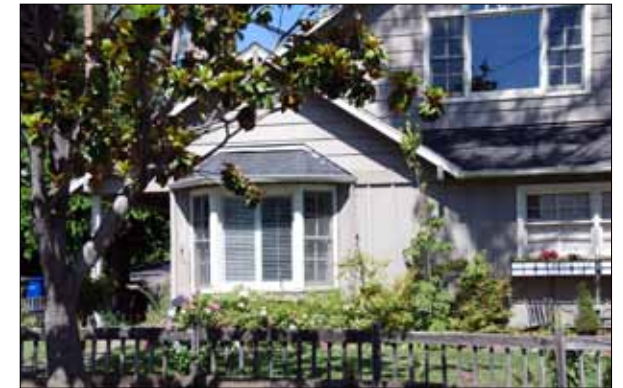
Matching the bay window roof material to the house is often a good way to integrate it into the home design
