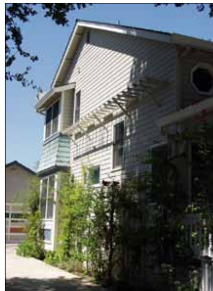
Horizontal elements such as trellises can be used to break up taller vertical walls.
