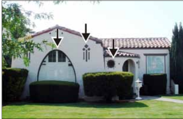
Shaped window, decorative tile and metal grilles
