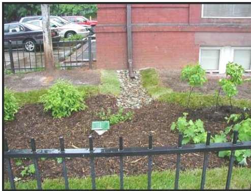
A Low-Impact Development Disconnected Downspout
