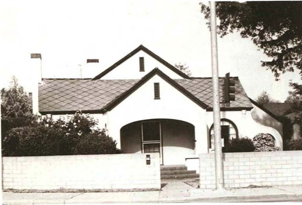
Photo from Sunnyvale Historic Inventory
