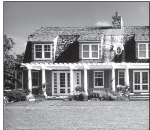
3.9.B Landscaped trellises can be used to add visual interest and integrate long elevations
