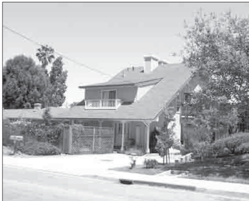
3.4.B Integrating second floors into a gable roof is one way to minimize two story building bulk
