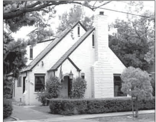
High quality textured stucco walls used on all walls and slate roofing used on simple gable forms give this home a unified design appearance
