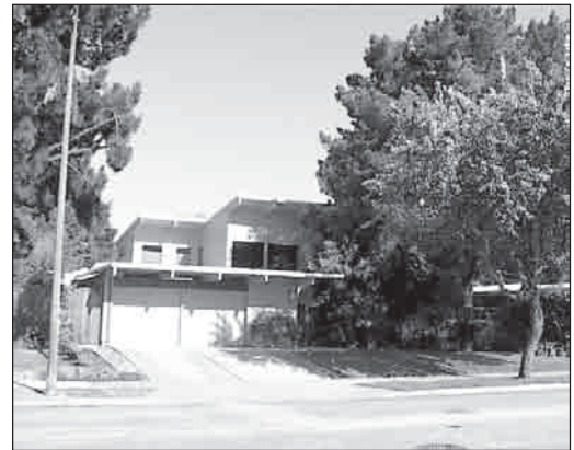
3.5.L Similar roof pitch and eave detailing on this Eichler home assist in unifying the second story addition
