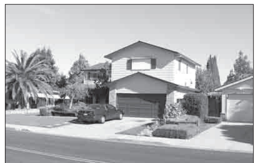
3.4.S Avoid second floors like this over garages unless stepped back substantially
