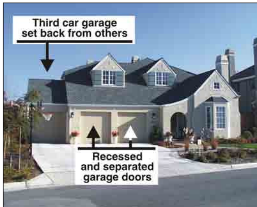
3.2.E Break up the mass of two and three car garages 3.2.F
