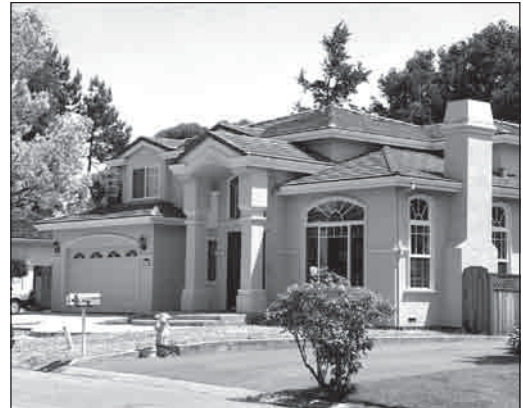
3.5.A Avoid complex roof forms like this
