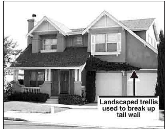
3.4.Q Projecting trellises and lattices can help to soften the appearance of tall wall areas
