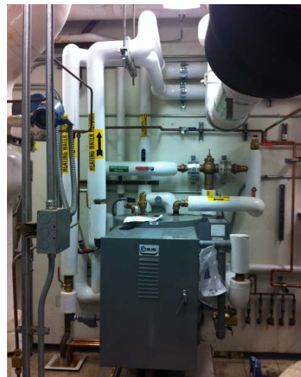
Building conversion from steam to hot water
