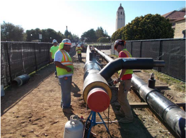
Construction crews install piping along Serra Mall
