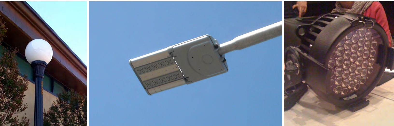
Photos: Lighting projects across campus work to improve energy efficiency. Left: Typical outdoor lighting fixture. Center: Pilot LED outdoor streetlamp. Right: High-efficiency LED stage lighting.
