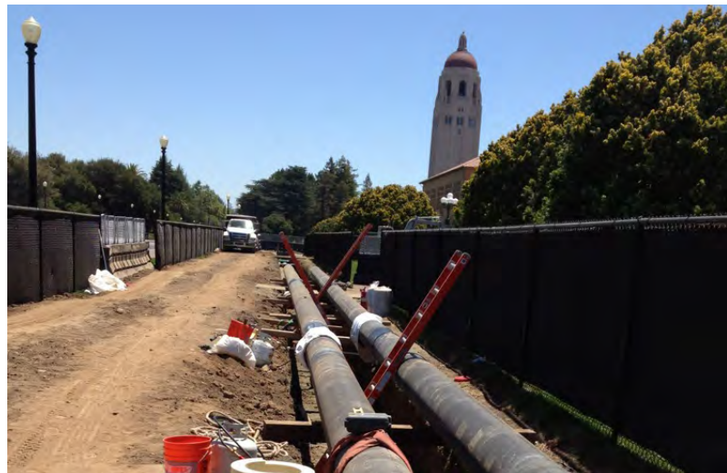
Photo: piping installation in progress along Serra Mall.
