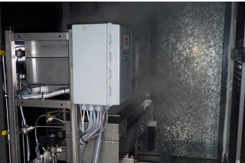
Photo: New high-efficiency ultrasonic humidifier in operation
