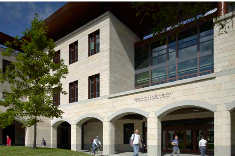
Photo: Yang & Yamazaki Environment & Energy Building (Y2E2)
