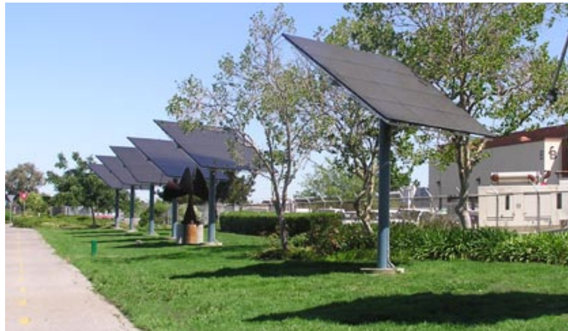
The photovoltaic panels installed along the frontage road at the MSC are “trackers”. They pivot to follow the sun—maximizing the amount of electricity they can produce each day.
