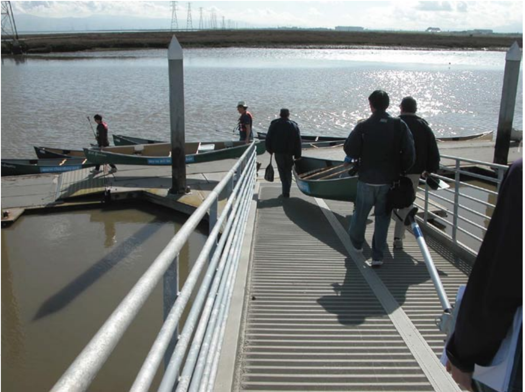
The boat dock at the Palo Alto Sailing Station meets very strict criteria established by the BCDC. It is designed to avoid harming the benthic organisms that live in the muddy area along the shore. Also, even when the tide is low it does not rest too long on the bottom as that would be viewed as "filling in the Bay".
