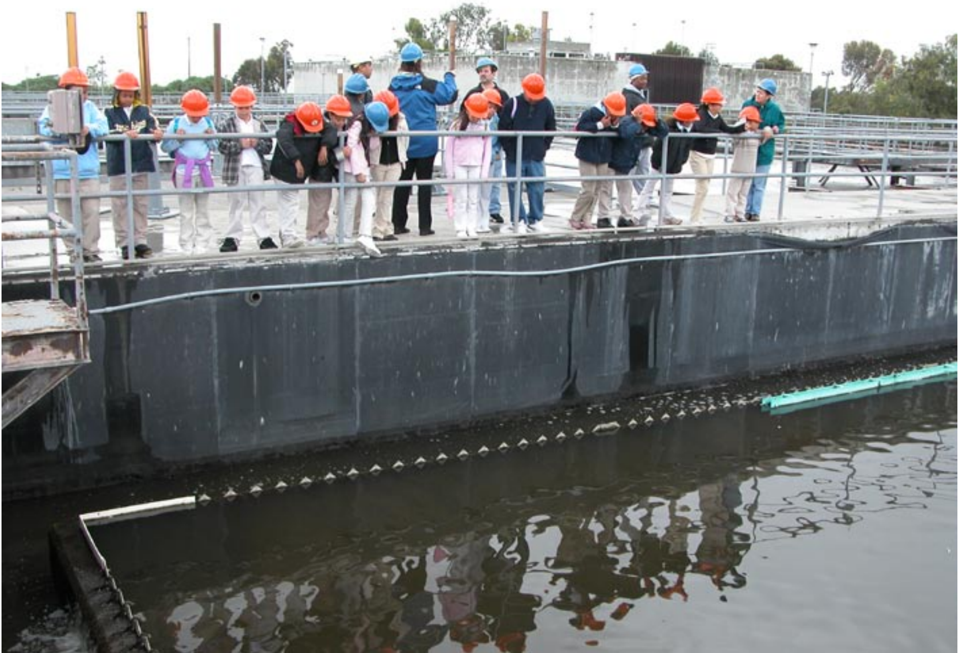
The Regional Water Quality Control Plant has been designed to remove most of the organic pollutants found in wastewater. The plant consistently removes 99 percent of these organic and solid pollutants which has gone a long way to restoring the health of the South Bay. Shown above is a school tour of the waste-water clarifiers. Also see "Thank you" letter from one of the tour participants in this chapter.
