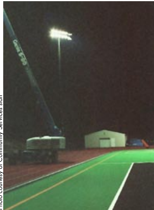
The new light field and security lights represent significant improvements in terms of energy efficiency, efficacy of field illumination, and reduction in glare and off site spill factors.
