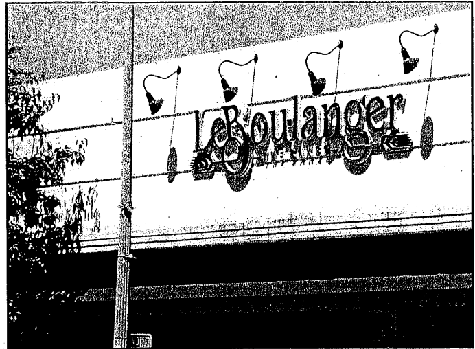
GUIDELINE 5.7.1. Building face signage of high-quality, individual letters, lit with wallwashing lights.
