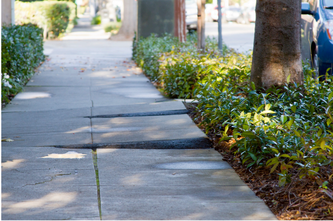
Figure 2-1. Asphalt is often the mediator in the continuous battle between roots and sidewalks.
