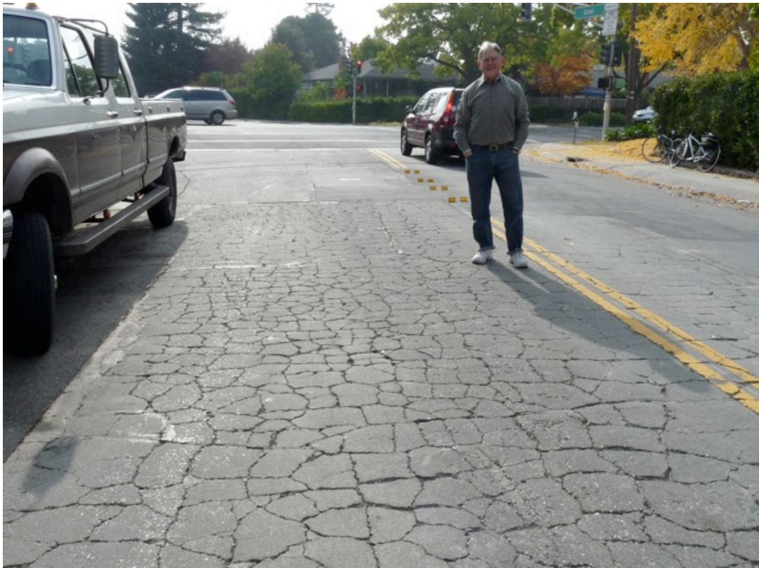
Figure 2-2. Street condition on Greer Road between Embarcadero and Channing, rated 38 on the PCI Index (“very poor to serious”).
