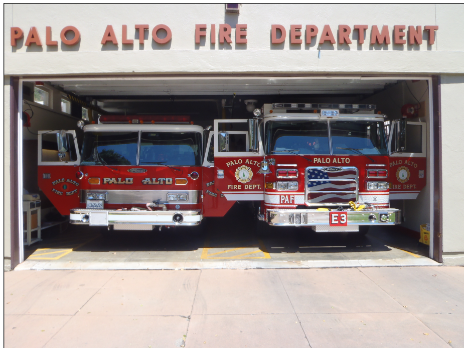
Figure 3-1. Palo Alto Fire Station 3 lacks sufficient space for modern equipment and does not meet current seismic standards. It was built in 1948 to codes that are now significantly out of date.
