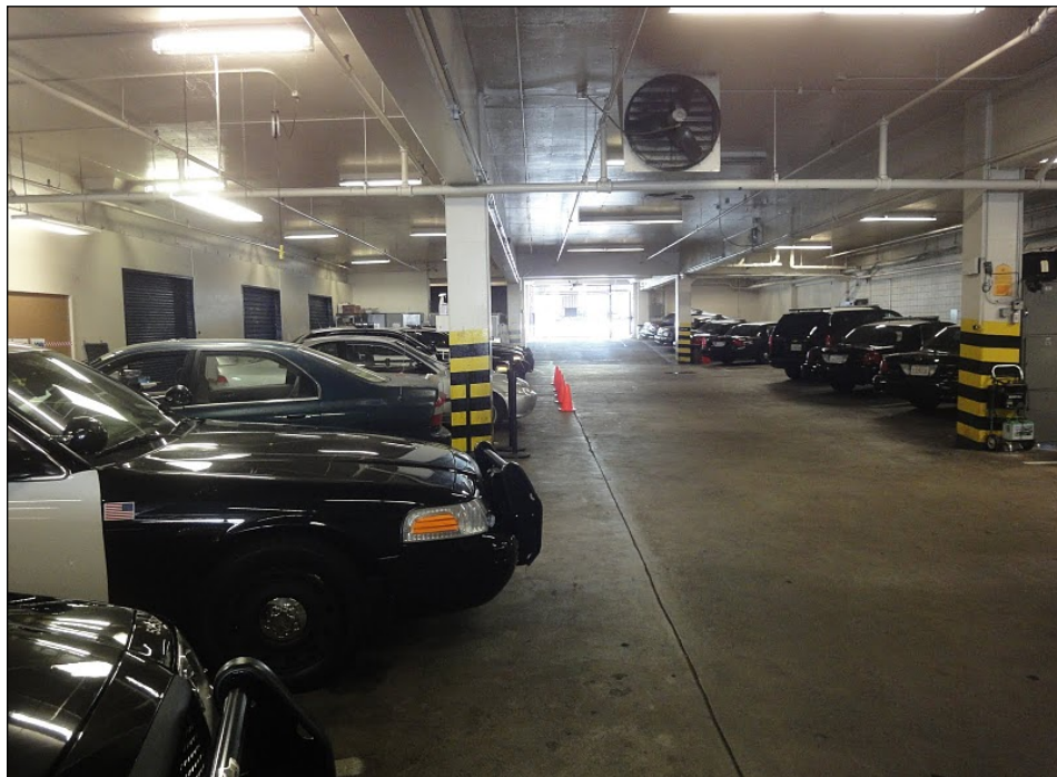
Figure 3-3. The Palo Alto Police Department garage is open at both ends and sits above the city public parking garage. Being so situated renders it extremely insecure, vulnerable to penetration or blasts from both outside and below. A more defensible design would have just one secured entry point located away from the vehicle fleet.
