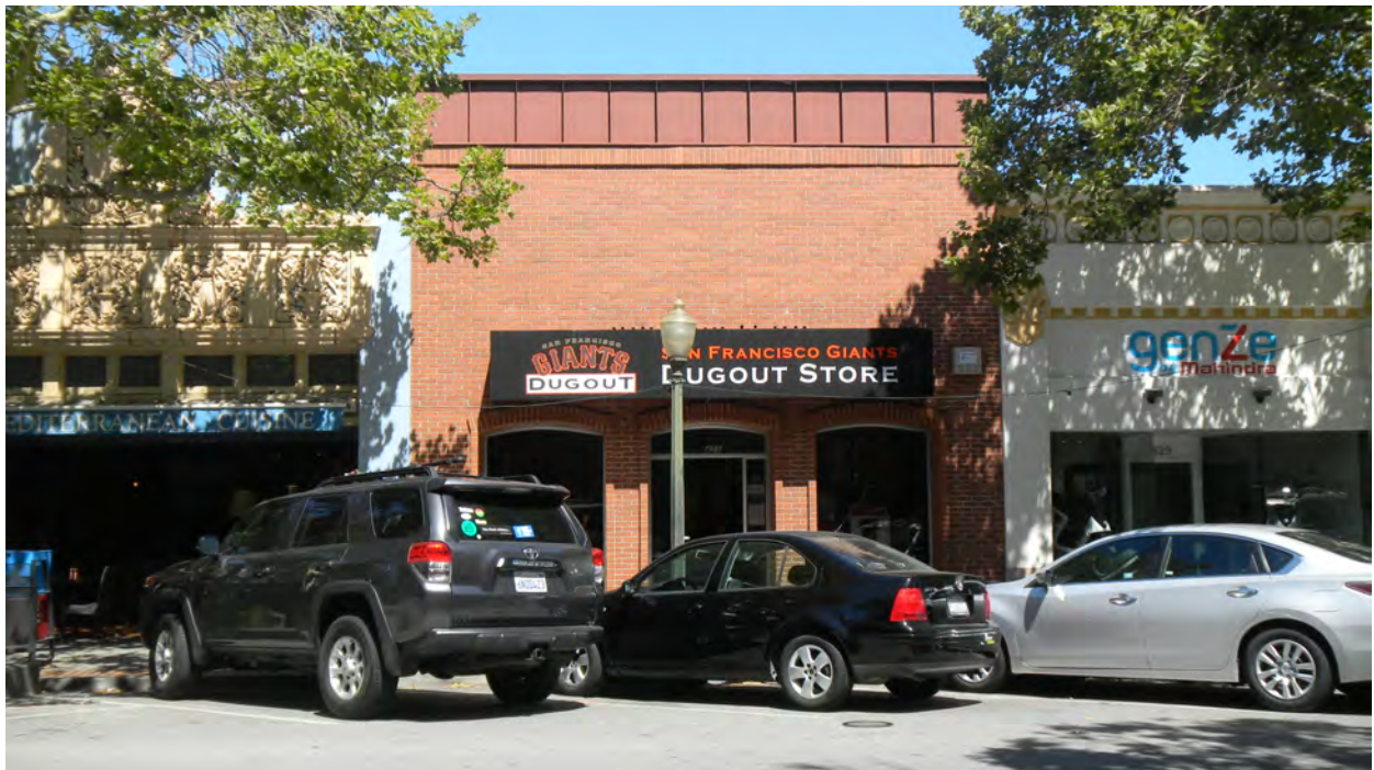
Fig.2 – 425 University Avenue – Front View Detail of front façade
