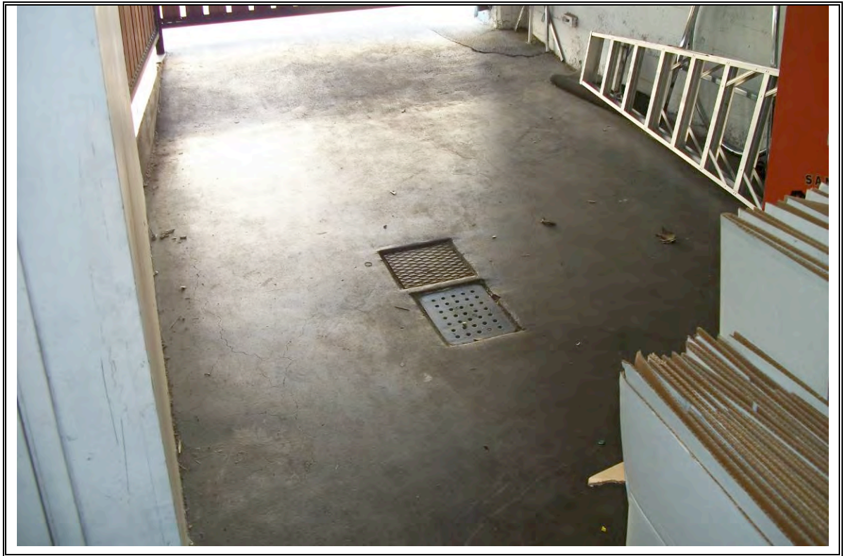
Photo No. 15: Concrete floor and storm drain in the parking space
