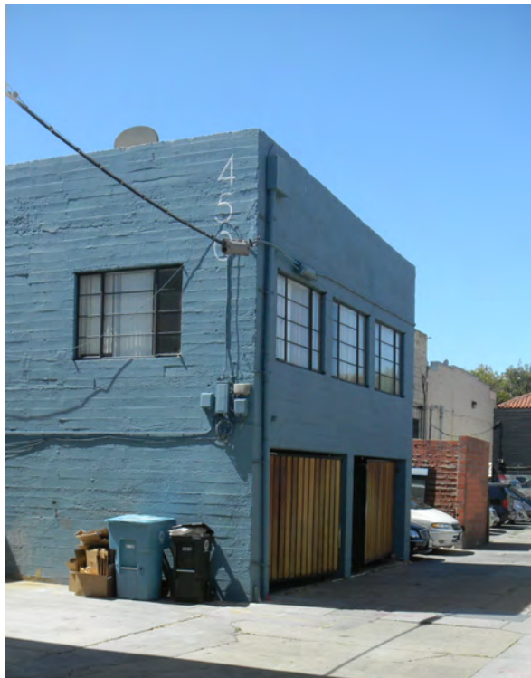
Fig.4 – 425 University Avenue – Rear View (from east)
