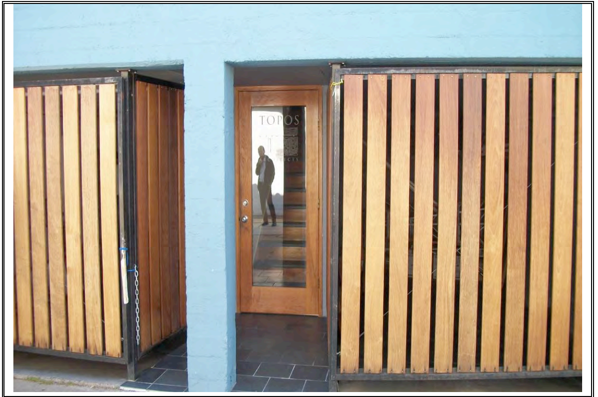
Photo No. 17: Entry door to the rear of the building and stairway leading to the 2 nd floor
