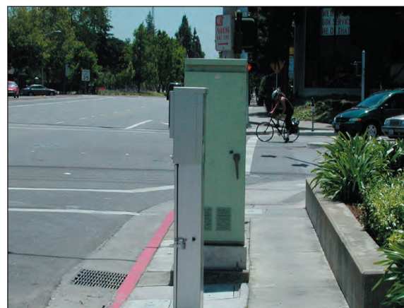
Figure 4.36: Example of landscaping and signal equipment further constricting an already narrow sidewalk.
