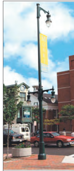
Figure 5.55: In a “combined” light fixture, both roadway and pedestrian fixtures share the same pole.
