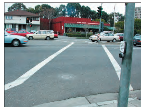
Figure 4.40: Crosswalks on El Camino have an average length of 104 feet. The distance increases where crosswalks are not perpendicular to the roadway.
