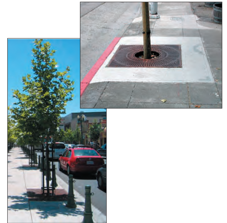
Figure 5.61: Tree grates and tree guards can add to the life of the tree and the aesthetics of the streetscape. The upper image shows a retrofit tree grate, while the lower shows new construction.
