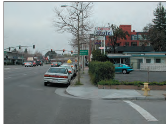
Figure 4.37: Example of diagonal curb ramp.
