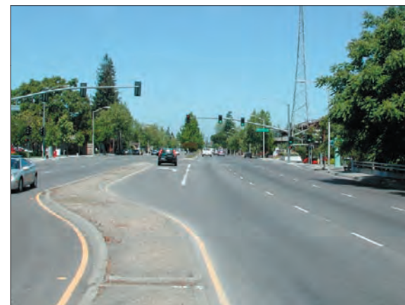
Figure 4.16: El Camino Adobe Creek (looking north).
