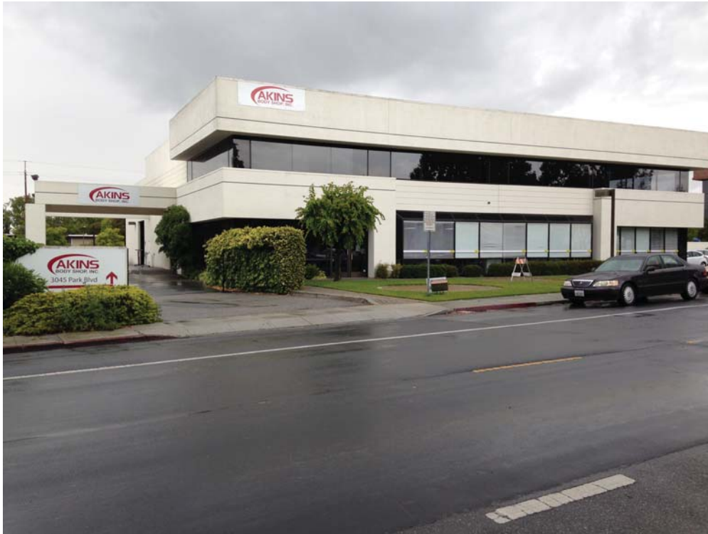
Photo 3: View of the 3045 Park Boulevard site from across Park boulevard.
