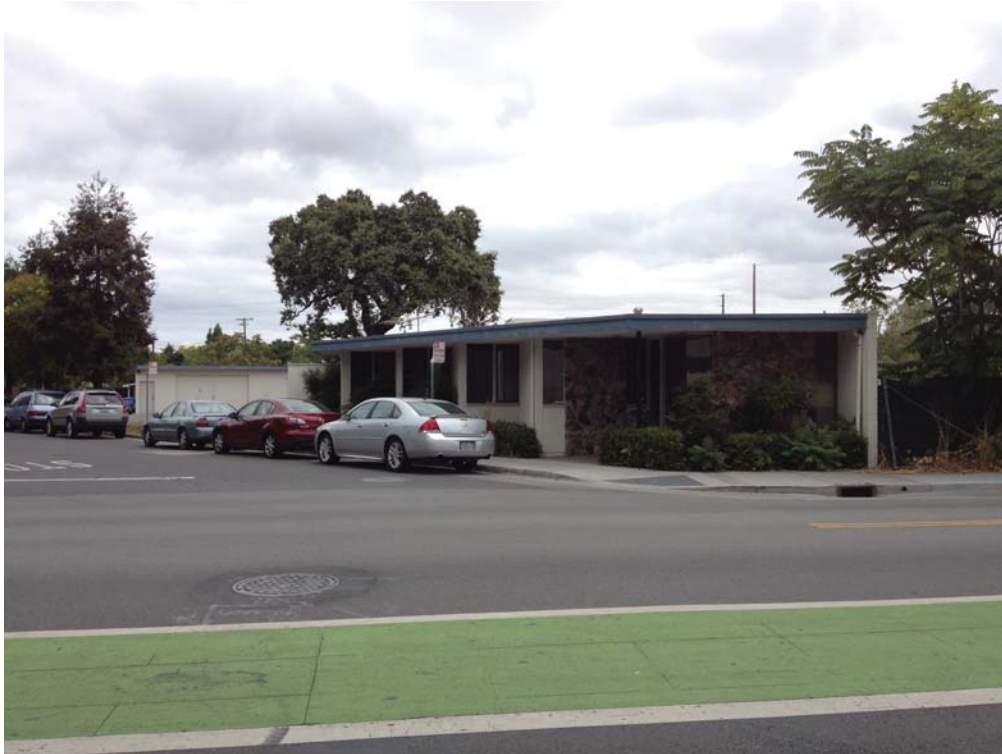
Photo 1: View of the 2747 Park Boulevard site from across Park Boulevard.
