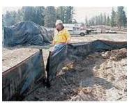
Upon inspection, it was determined that this silt fence was installed incorrectly.
