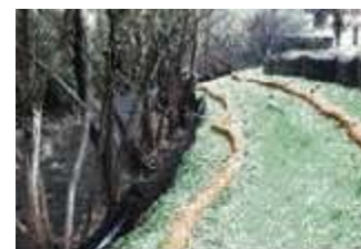
Silt fence and fiber rolls must be removed before acceptance of the contract unless other arrangements have been made with the District Maintenance unit
