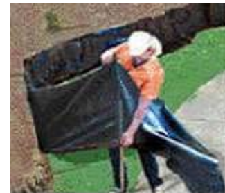
Silt fence must be removed and properly disposed of before acceptance of the contract.
