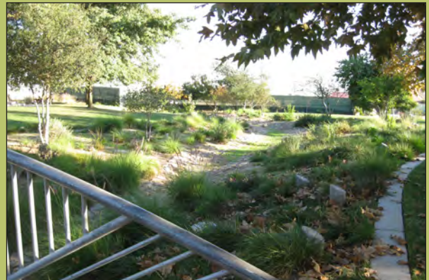
PICTURED: A vegetated channel, a green infrastructure feature, helps to naturally manage water at the park. (Source: EPA)
