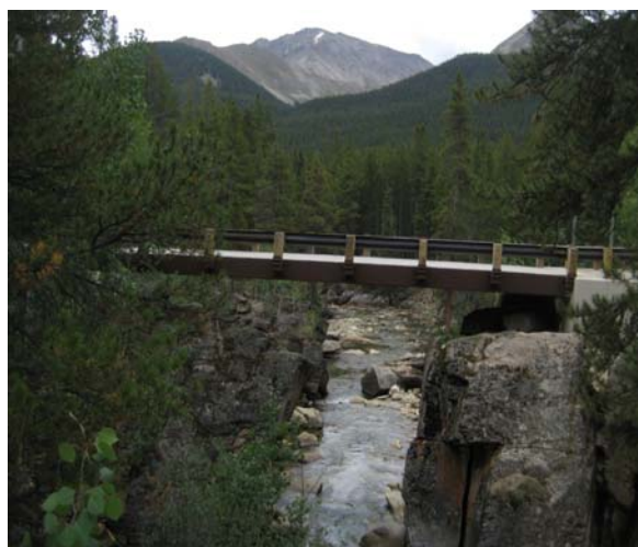
North Lake Creek Bridge Replacement, Pike-San Isabel NF, CO
