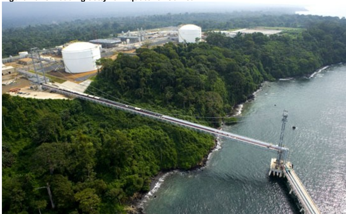
Figure 13: Offloading Jetty for Equatorial Guinea
