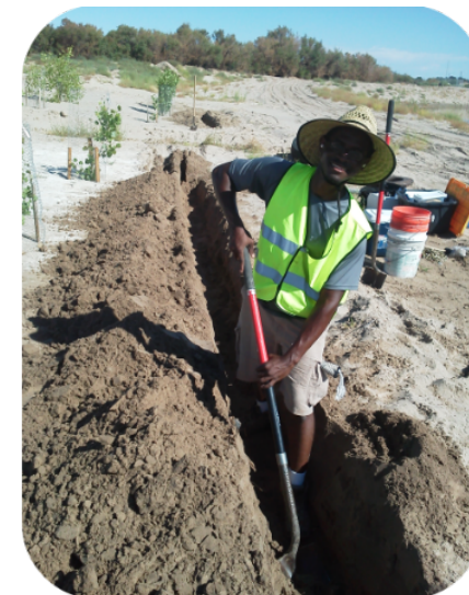
Drainage Pipe Installation
