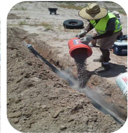
Drainage Pipe Installation
