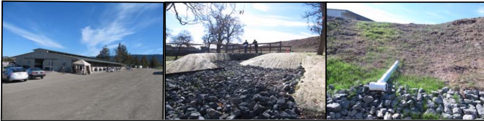
Left to right: building (20,000 sq. ft 2 ) with retention basin design; percolating section of the basin; and white, hillside drain directing storm water runoff into retention basin.
