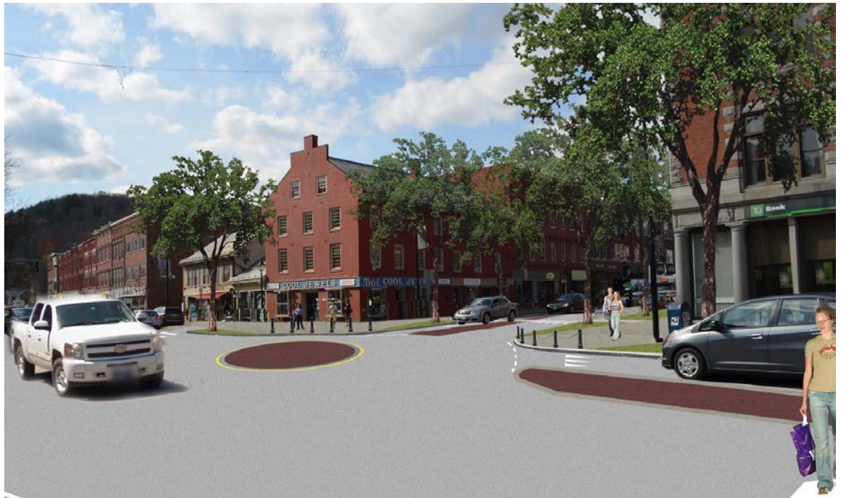
Figure 41: Design option for a mini-roundabout at the intersection of State Street and Main Street.
