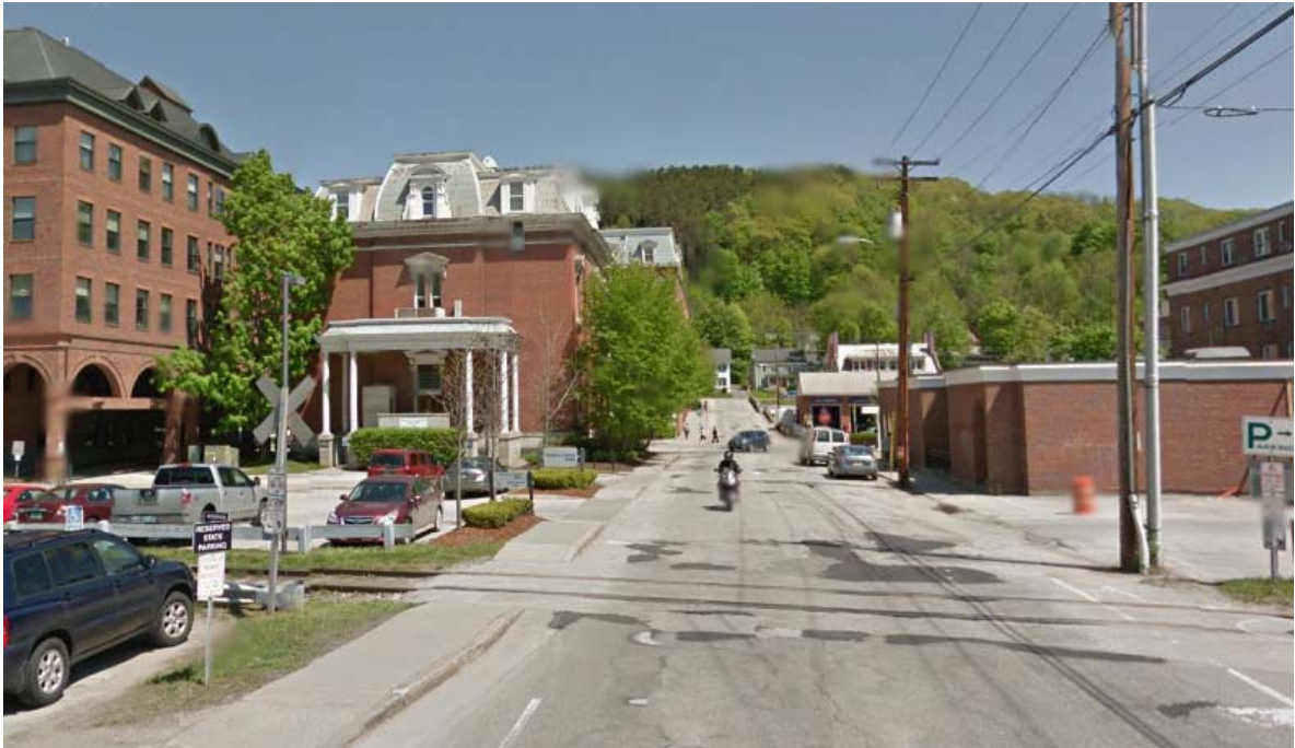
Figure 36: Current conditions on Taylor Street.
