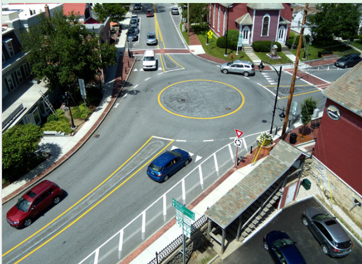
Figure 43: Mini-roundabout in Manchester. Photo courtesy of Stantec.
