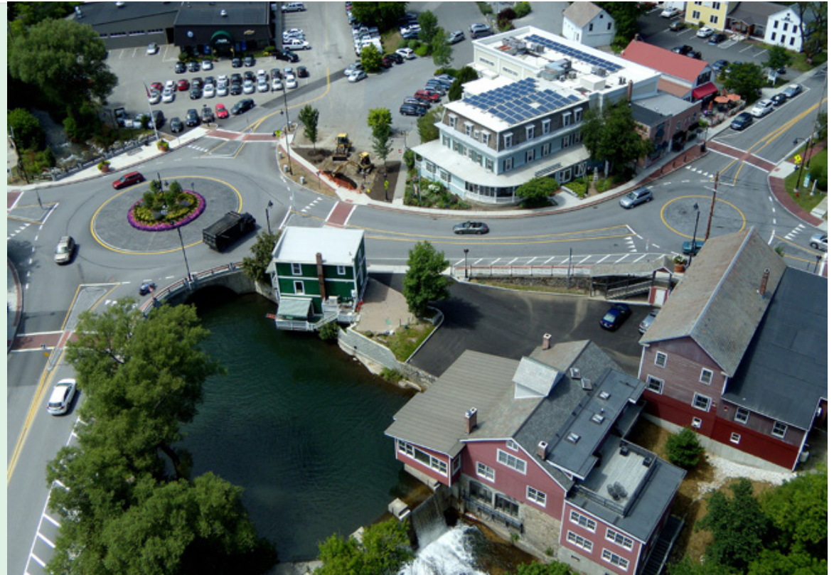
Figure 42: Single-lane (left) and mini- (right) roundabouts in Manchester, Vermont. Photo courtesy of Stantec.
