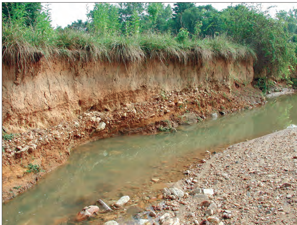
Figure 9. Section of unrestored Minebank Run stream channel in Cromwell Valley Park downstream from Interstate 695 near Towson, Maryland. (Photograph by Robert J. Shedlock, U.S. Geological Survey)
