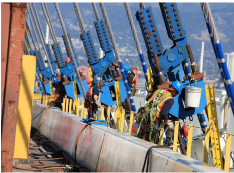
TENSION SUSPENDER ROPES
