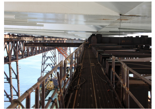
DECKS LIFT UP FROM TEMPORARY SUPPORTS
