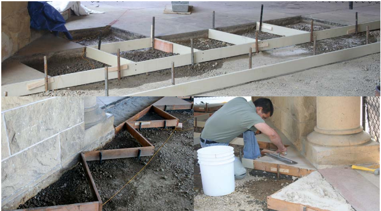
Main Quad - Paver Renovation Project
