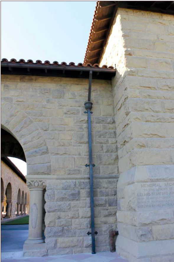
Main Quad - Drainage Improvements
