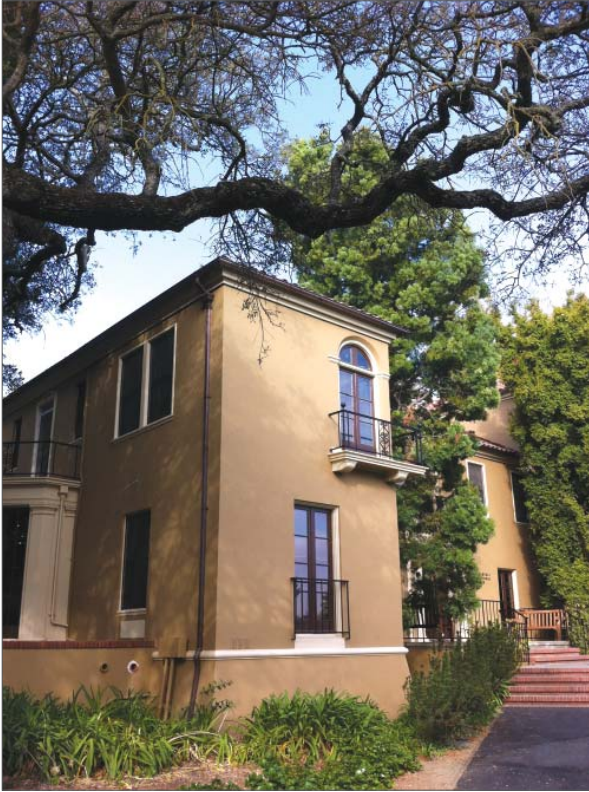
Bechtel International Center - Exterior Renewal
