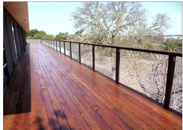
Center for Advanced Study in the Behavioral Sciences (CASBS) - Deck Replacement
