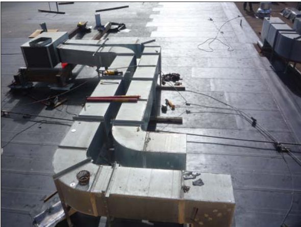
Stanford Auxiliary Library - Roof Replacement
