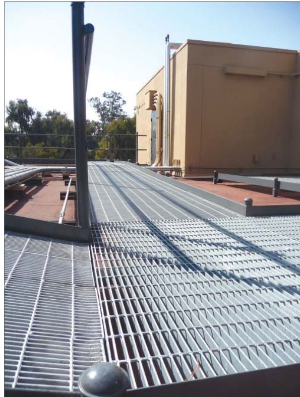
Forsythe Data Center - Roof Cat Walk Extension
