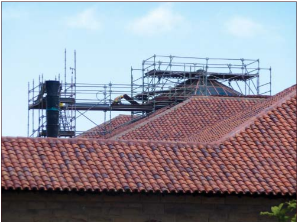
McClatchy - Roof and Skylight Renewal
