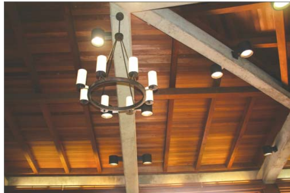
Faculty Club Main Dining Area - Lighting Energy Retrofit
